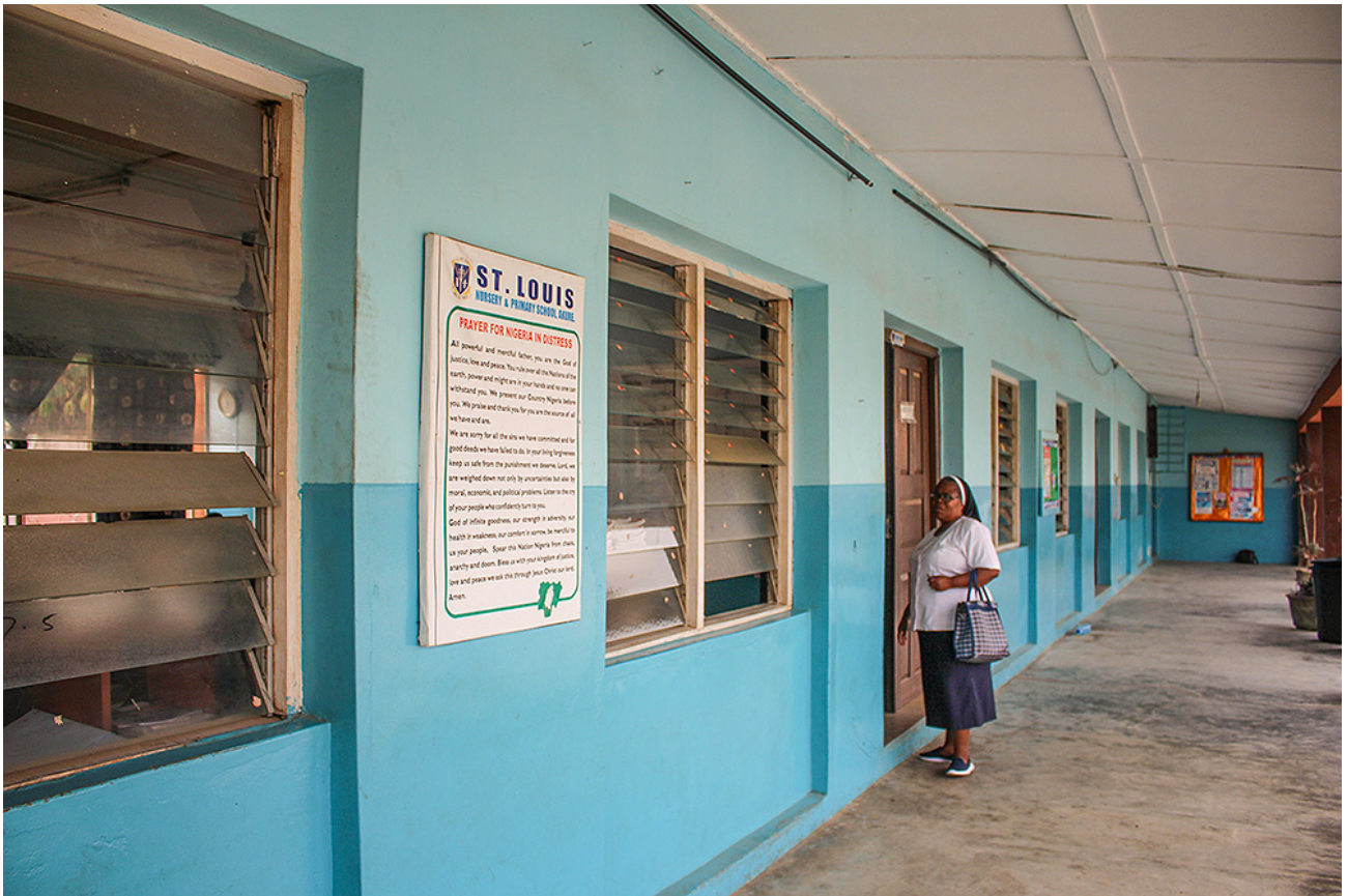
The grade 1 classroom block at St. Louis Nursery and Primary School, run by the Sisters of St. Louis in Akure, Nigeria (GSR photo/Valentine Benjamin)
