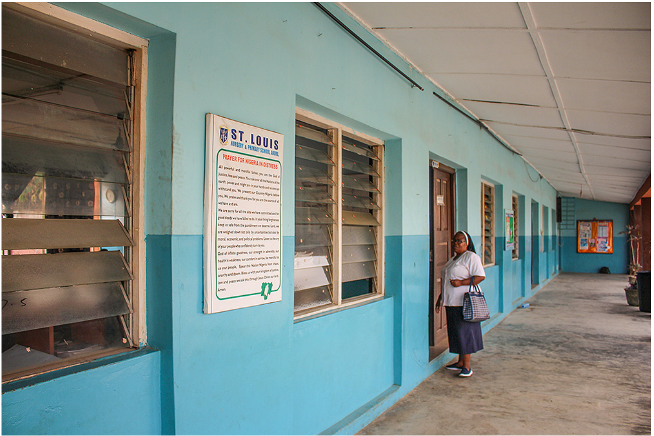
The grade 1 classroom block at St. Louis Nursery and Primary School, run by the Sisters of St. Louis in Akure, Nigeria (GSR photo/Valentine Benjamin)
