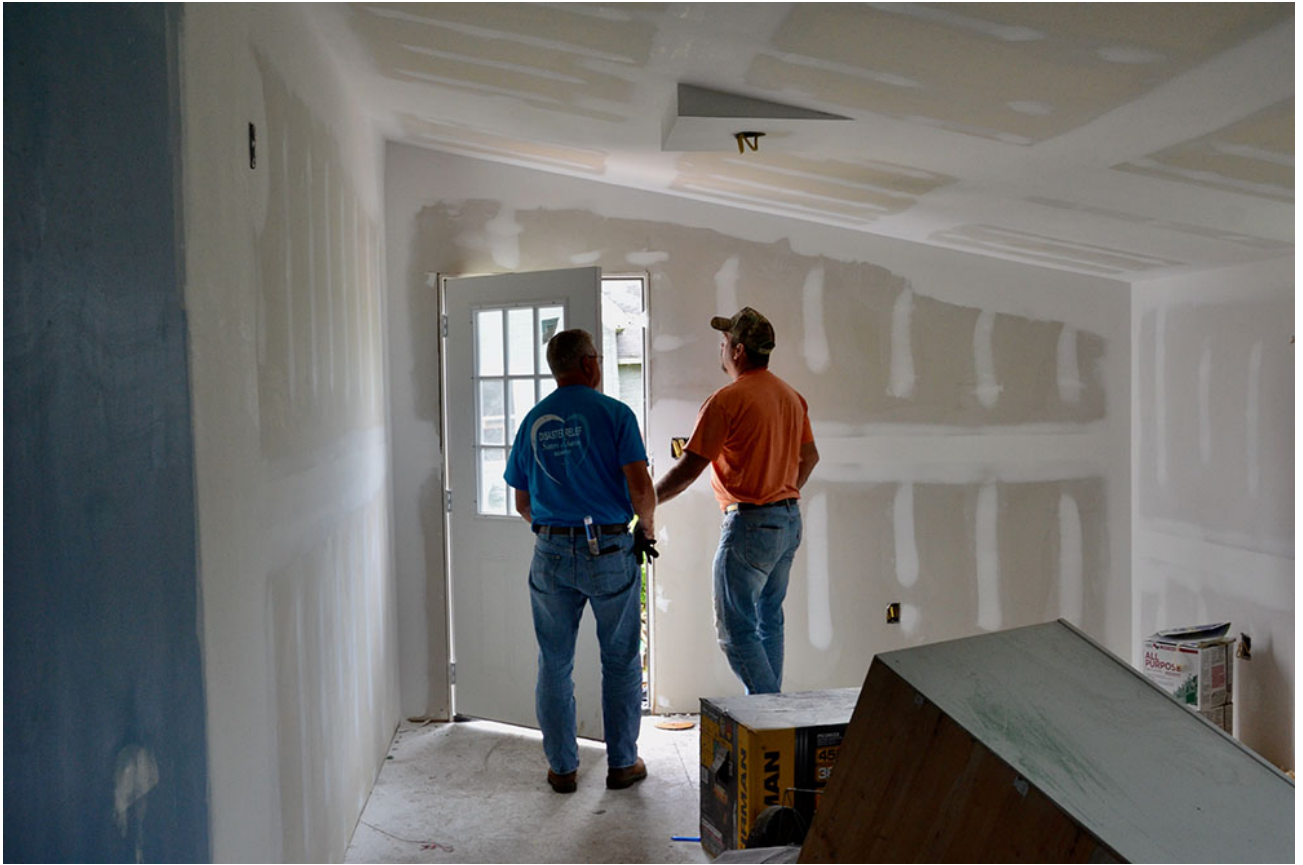
David White, left, and Ronnie Mattingly check out a leaky door May 23 at a house in Mayfield, Kentucky, damaged by a tornado in December. (GSR photo/Dan Stockman)
