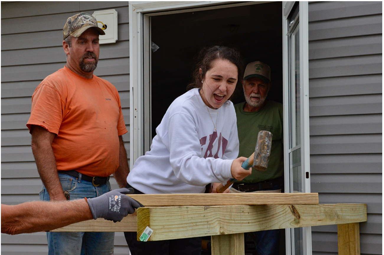
Ronnie Mattingly, left, and Jude Leake watch Lizzi Seyle try the sledgehammer May 23 as the disaster recovery team works on a home damaged by a Dec. 10 tornado in Mayfield, Kentucky. (GSR photo/Dan Stockman)
