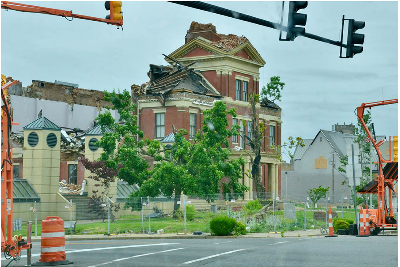
• What is left of the Graves County Courthouse in downtown Mayfield, Kentucky, on May 23 (GSR photo/Dan Stockman)
