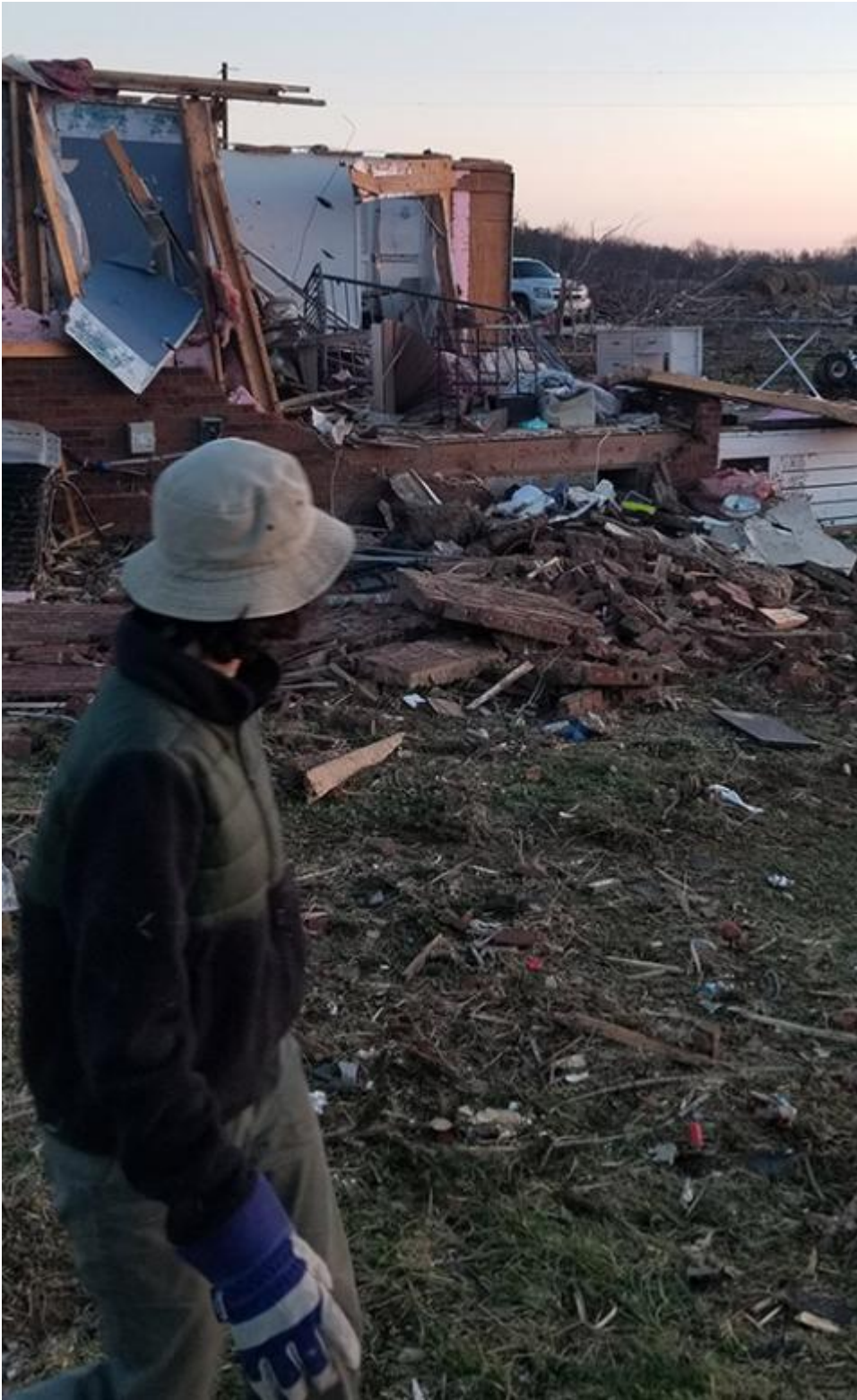
Julia Gerwe surveys damage caused by the Dec. 10, 2021, tornadoes in western Kentucky. (Courtesy of Erica Watts)
