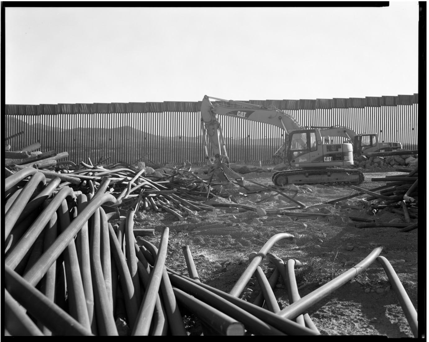
Outside Forrest, Arizona, in the last weeks of the Trump presidency, pieces of the old wall are thrown away as a new wall is built. (© Lisa Elmaleh)
