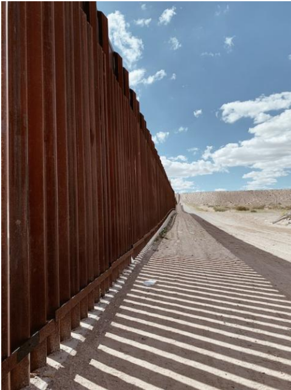
The border wall in Anapra, New Mexico (Celine Reinoso)
